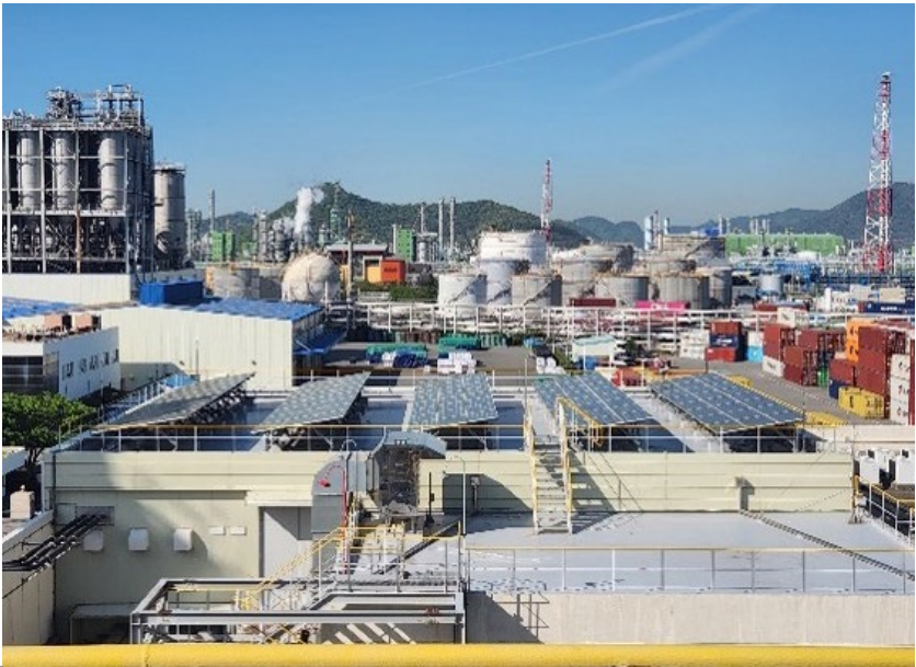
Rooftop solar panel installation
